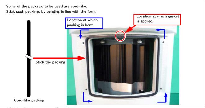
Fig.5-6: Sticking the cord-like packing
