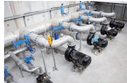
Sewage treatment plant
