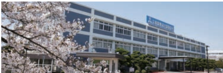
Mitsubishi Electric Nagoya Works
